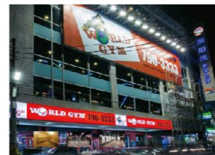
Fengshan Shopping Mall, Kaohsiung, Taiwan
